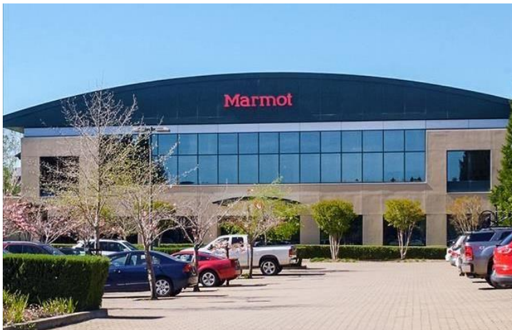
Marmot Headquarters on State Farm Drive in Rohnert Park.
