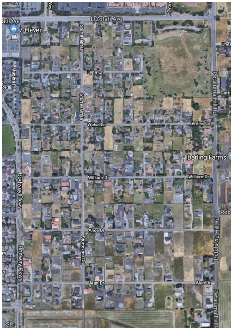
Aerial of Canon Manor Subdivision
